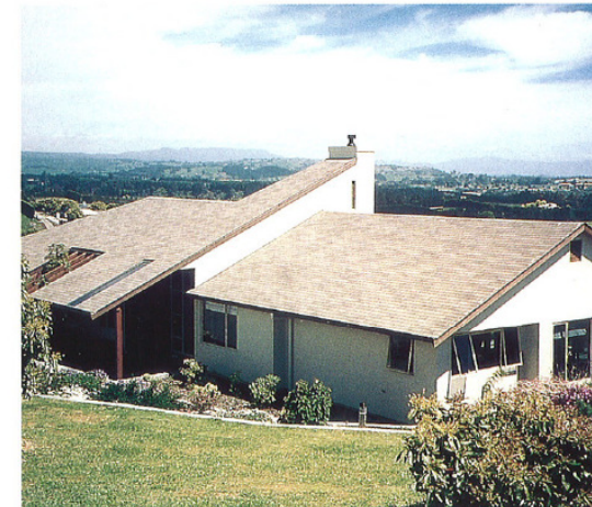
Vent near chimney
