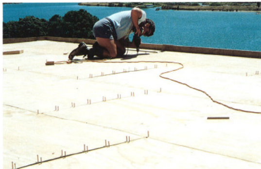
Note: Staggered sheets and screw fixing.
