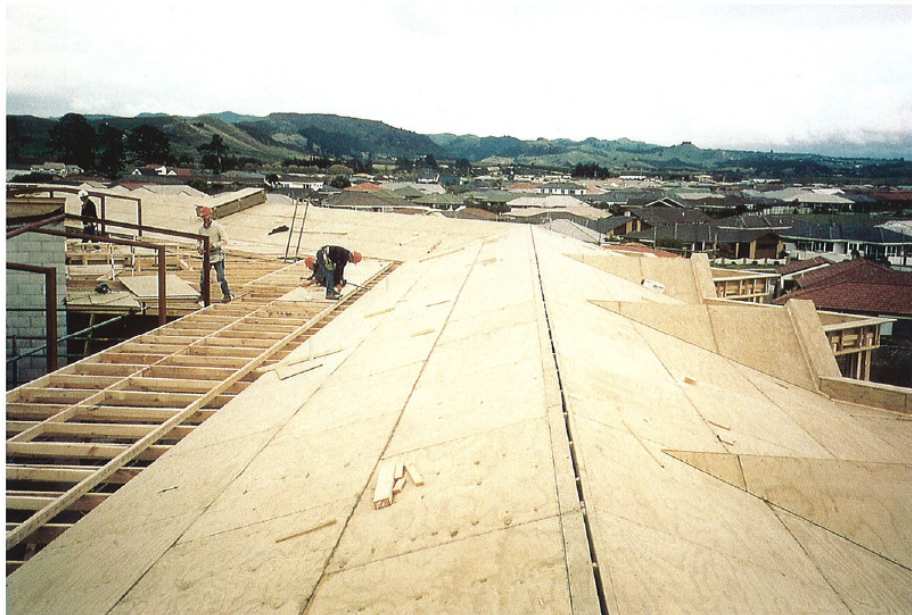
Note ridge vent
